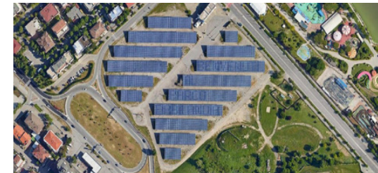
REMIMI, ITALY 1.8 MWp
