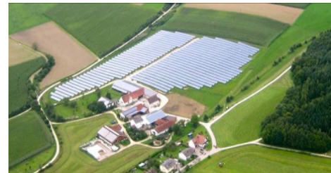
WOLPERSTETTE, GERMANY 2.2 MWp
